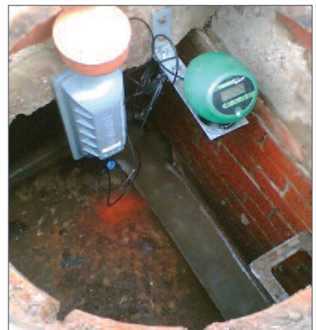
IMP MONITORING IN A CSO CHAMBER
