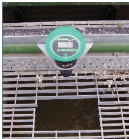
IMP CONTROLLING GATE HEIGHT
